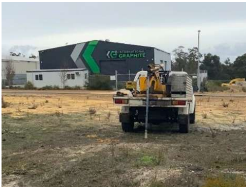
Left: Geotechnical drilling on site.
