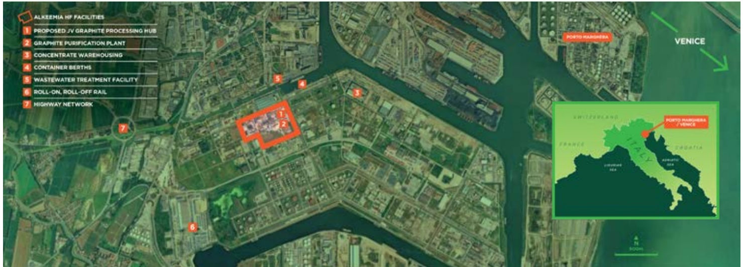
Figure 3. The Alkeemia site at Porto Marghera, Italy.
