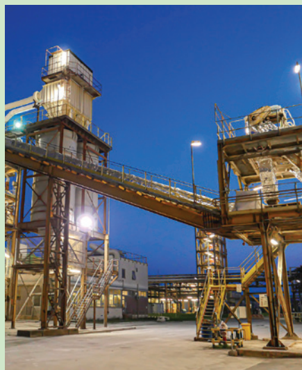
Figure 20: Alkeemia's hydrofluoric acid production platform at Porto Marghera.
